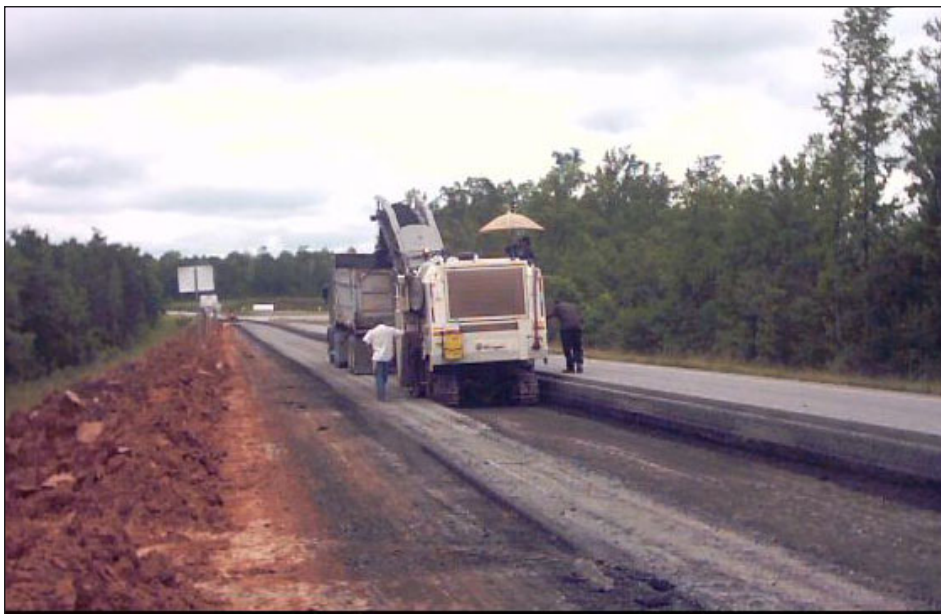
Reconstruction in progress for installing eight structural test sections
