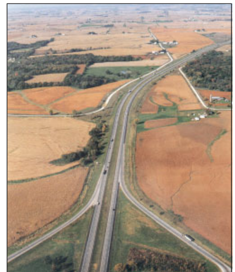
2002 Perpetual Pavement Award winner Interstate 80 in Cedar County, Iowa. The pavement has withstood 40 years of freeze-thaw cycles with flying colors.
