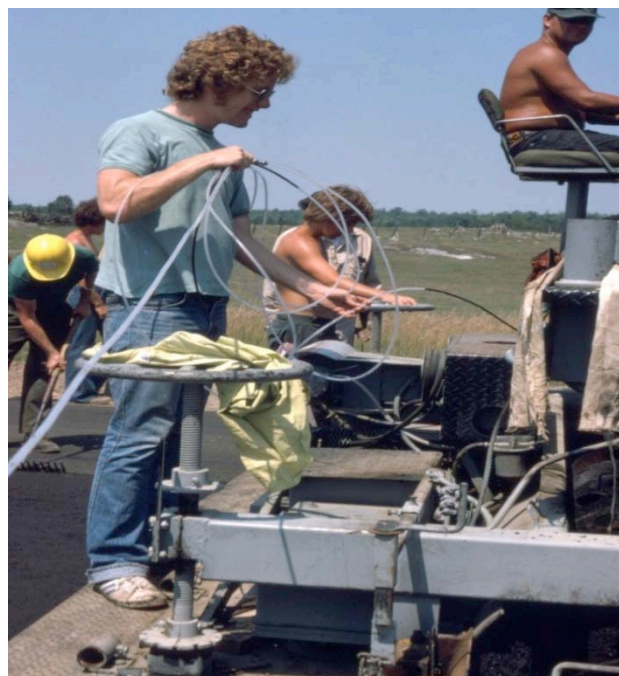
Figure 8: Sampling of fumes on the paver
