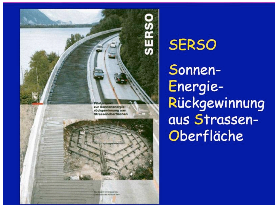
Figure 10: Sun energy recovery on Bern by-pass A1/6/12
