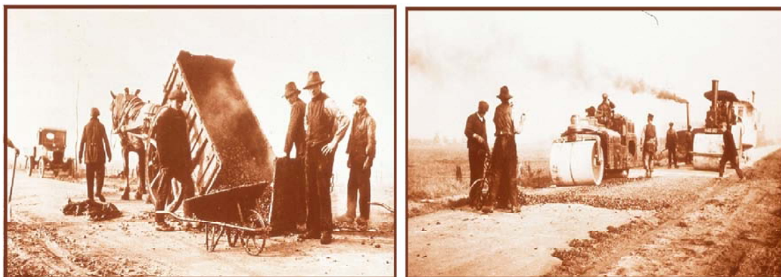
Figure 5: Early Pavement Construction & Figure 6: Motorized Pavement Compaction
