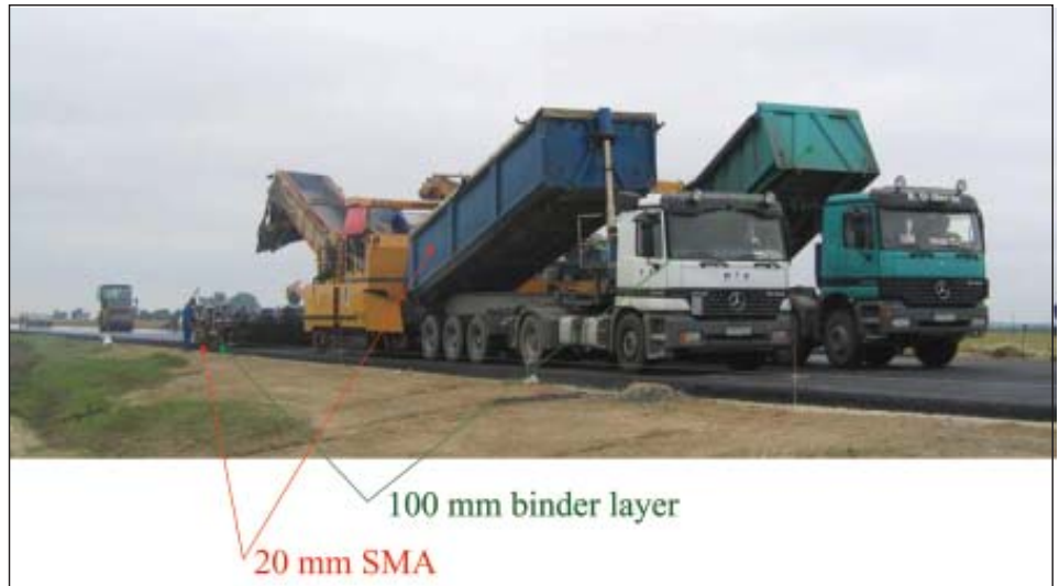
General view of the Compact-asphalt paving train
