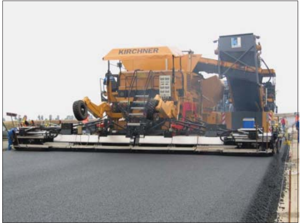
Mat behind the paver consisting of binder course and SMA
